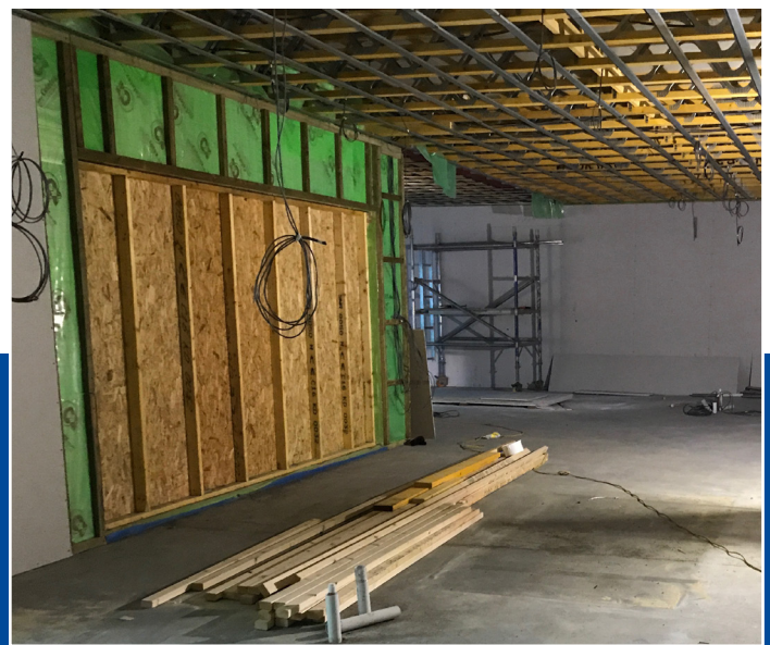
Internal finishes were safely installed in front of the CDM System.
