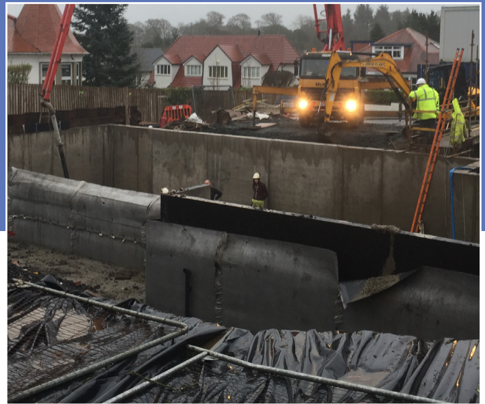
Newton 109-LM and 410 GeoDrain protect the external walls.
