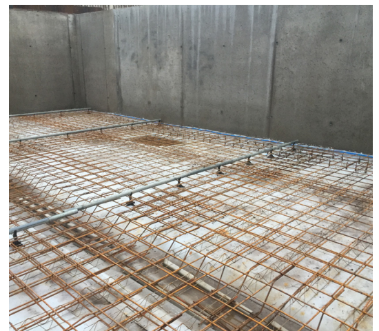
403 HydroBond provided protection beneath the slab.
