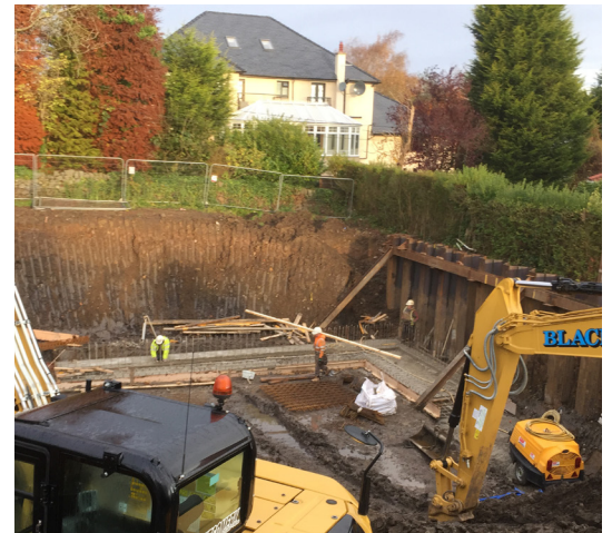
Extensive excavations were made for the new build.
