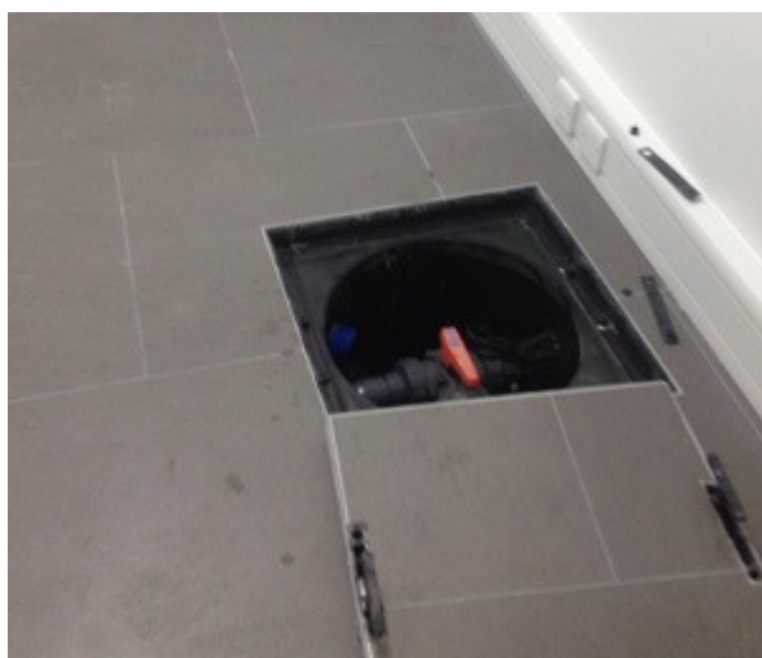
Four Titan-2 sump chambers pumps provided plenty of drainage.
