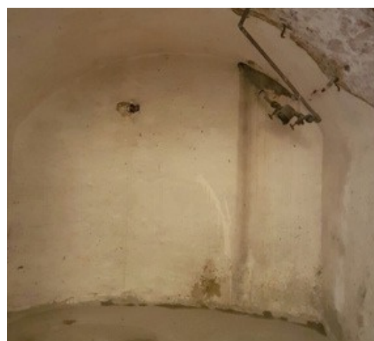
The original render was allowing in multiple leaks.
