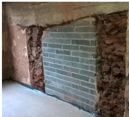
Partition wall to ensure continuity of waterproofing.
