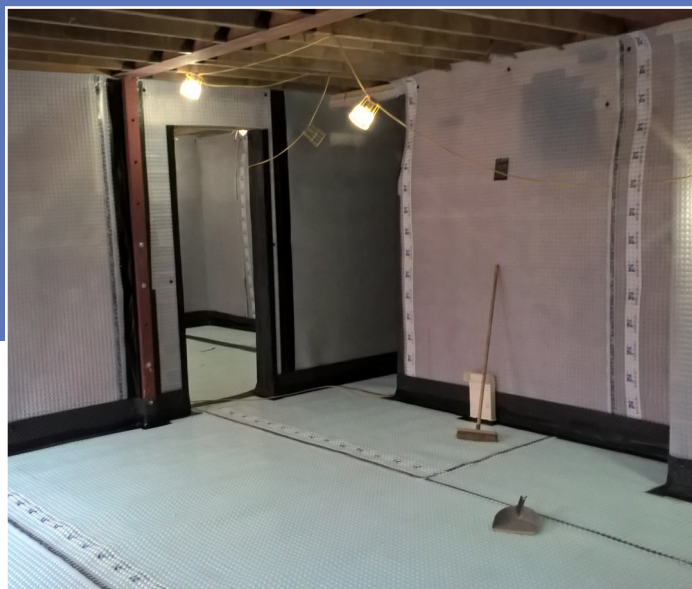
Drainage membranes to the floor and all internal walls.
