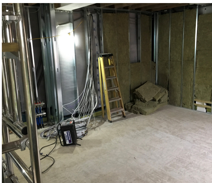
Installation of timber framed walls and insulation.
