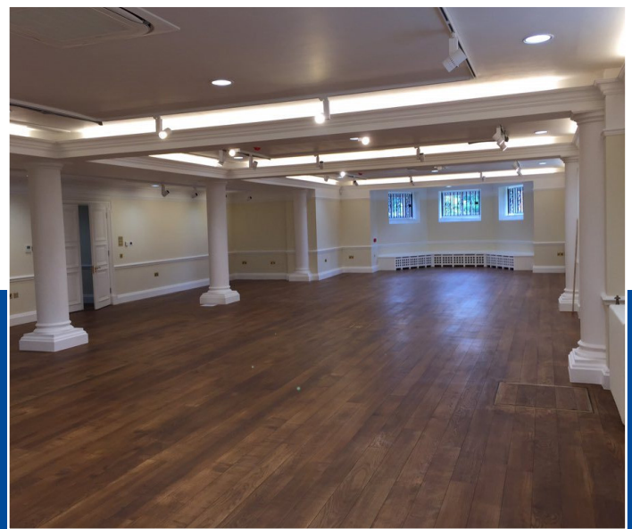
The completed project.
