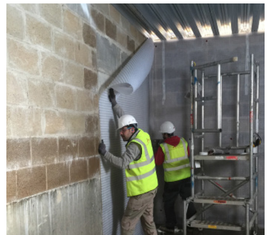
Newton 508 installed to the new extension walls.
