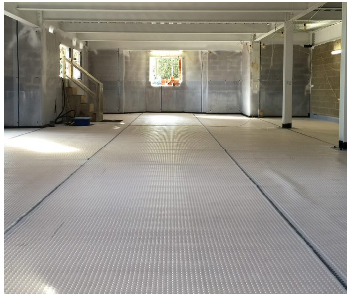
65mm of screed applied as a finish to the floor.
