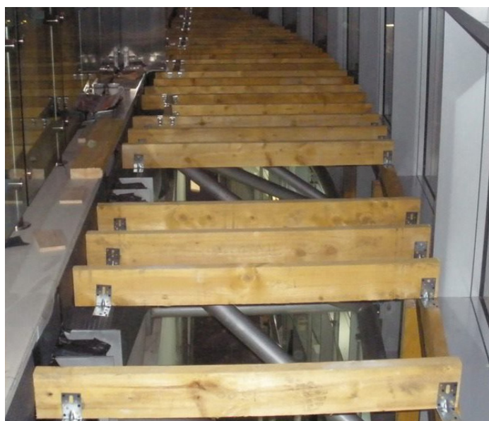
A new internal timber floor, wall and deck structure was required.
