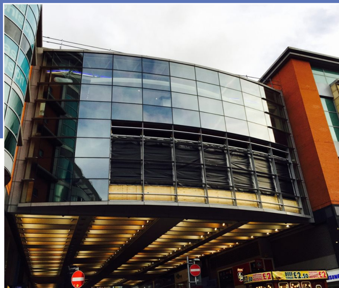
The digital screen was recessed into the building and fully weatherproofed.
