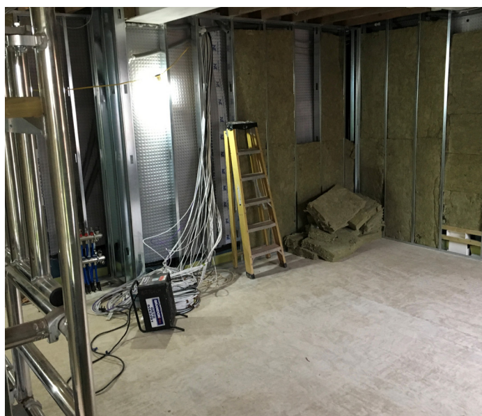
Installation of timber framed walls and insulation.
