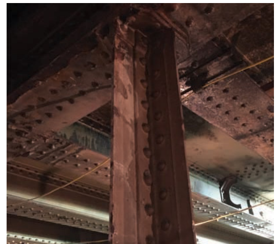
Steel beams supports the steel and concrete basement
