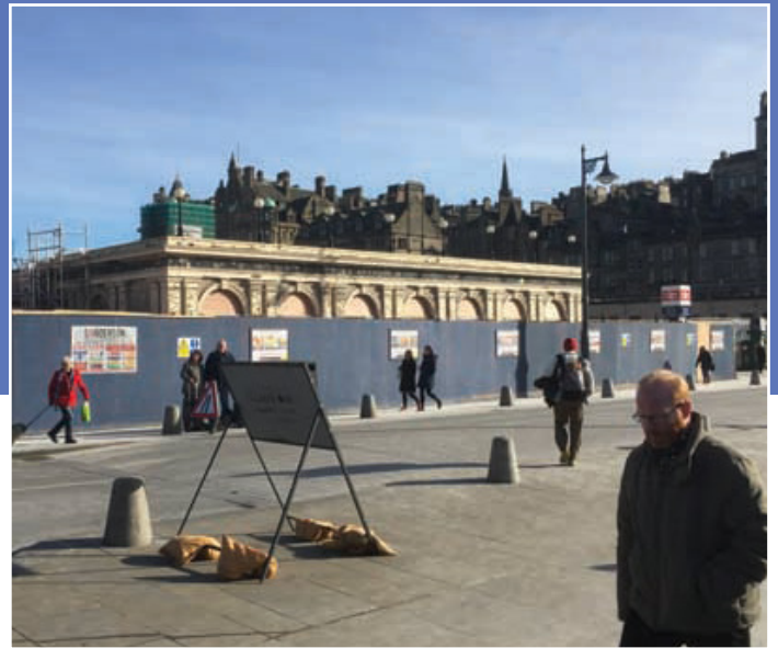
The busy road was one of the main sources of water ingress.
