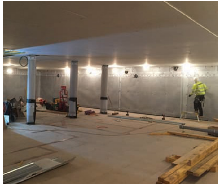
A new structure within the building was required.
