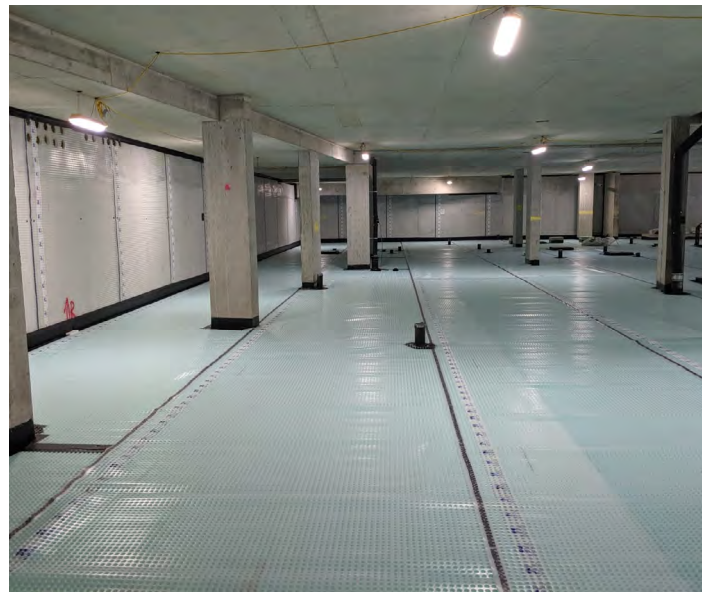
The full installation was an extensive basement waterproofing system.
