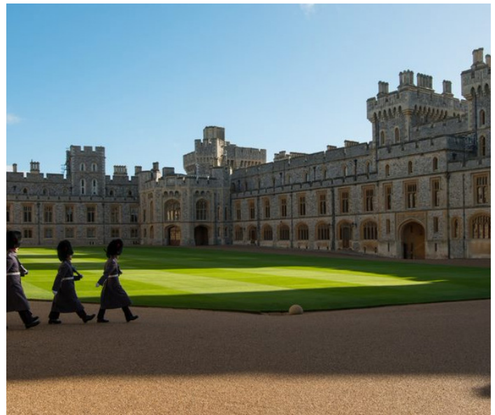
Issues with both rising and penetrative damp at the castle were resolved.
