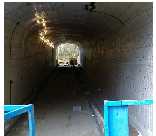
Newton 508 membrane lined the entire tunnel
