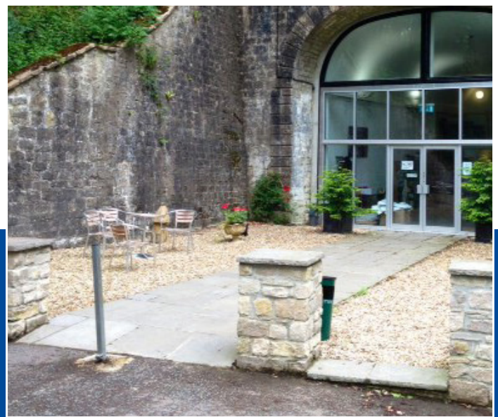
The exterior of the tunnel after completion.
