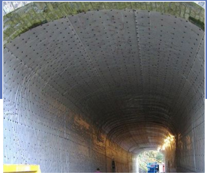
Application of Newton 508 Mesh to the tunnel walls.
