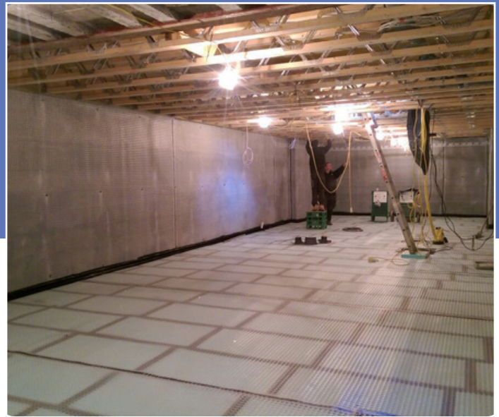
The system was installed rapidly and efficiently.
