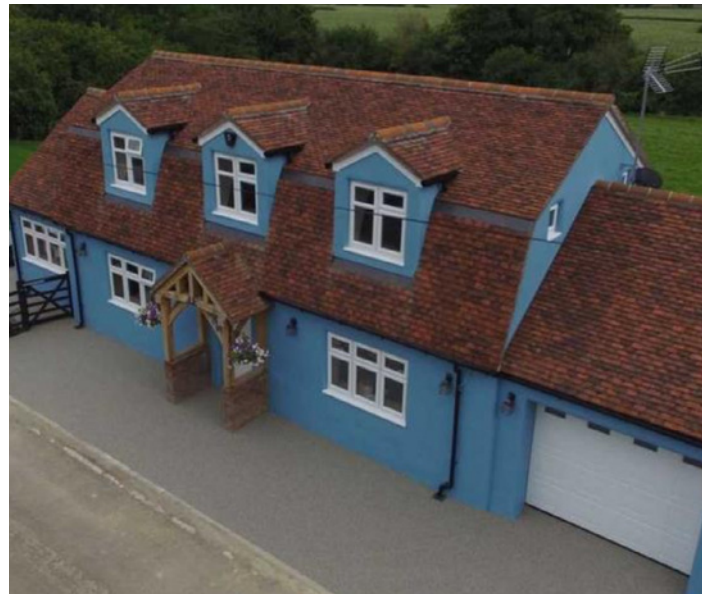
The waterproofing was for the basement of this new build residence.
