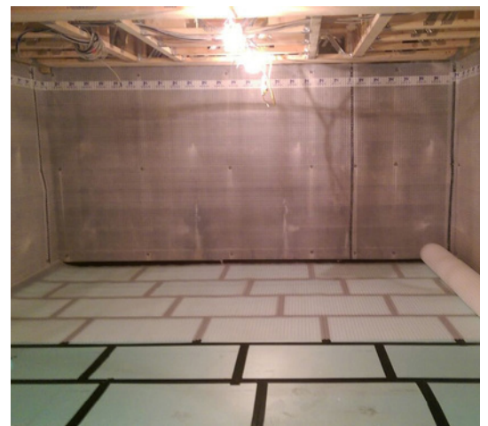
Installation of the failsafe Newton CDM System.
