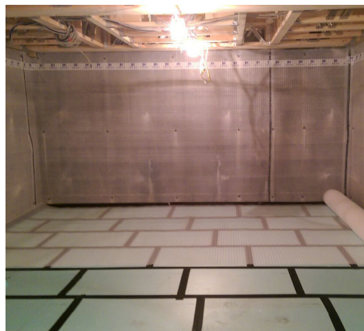
Installation of the failsafe Newton CDM System.
