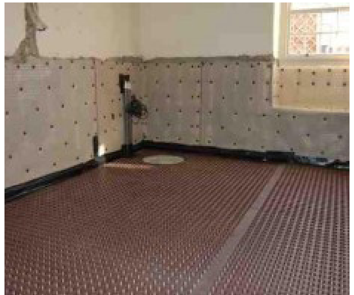
Newton System 500 was applied internally to protect from flood ingress.
