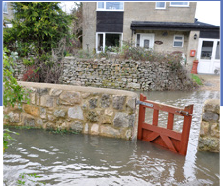
Major flooding in 2012 saw up to 800mm of water engulf South Hinksey.
