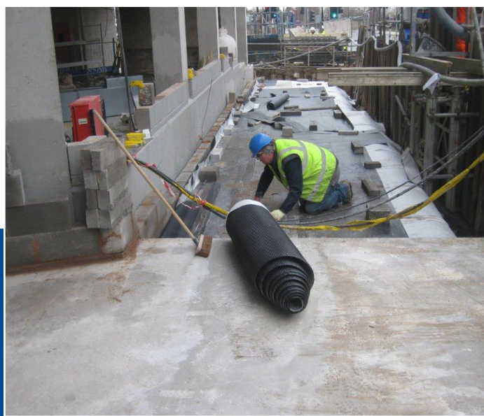
Newton 101F applied to the outer face of construction joints.
