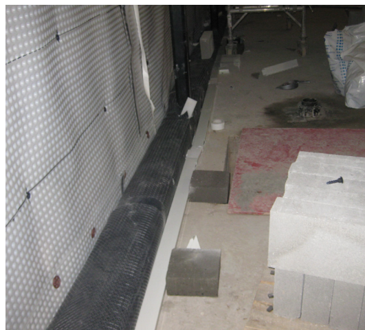
Newton System 500 was installed to protect from water ingress.
