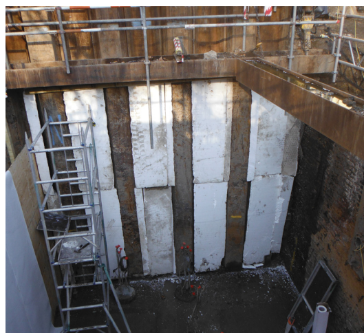
The deep, piled walls of the area to be waterproofed.
