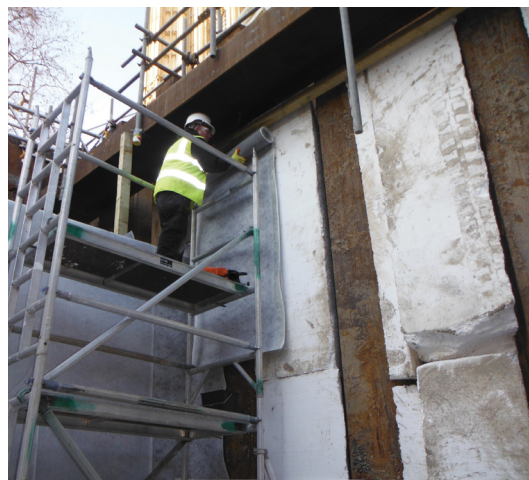
Applying 403 HydroBond directly to the piles.
