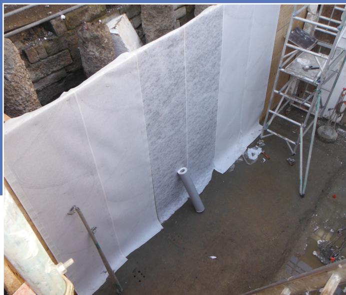
Newton 403 HydroBond is quick to apply in long sheets of membrane.
