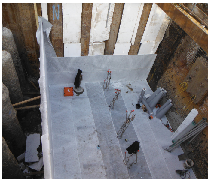
The membrane was used to create a complete waterproof envelope.
