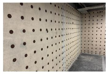
Laminated boards must be fixed to the wall with a mechanical fixing at each side of the board, to the upper half of the board, so that the laminated board does not come apart and block exits during a fire. This is a requirement of UK building code. Ensure that the mechanical fixings are either above the membrane height or where fixed through the membrane, above the expected height of moisture within the wall.
