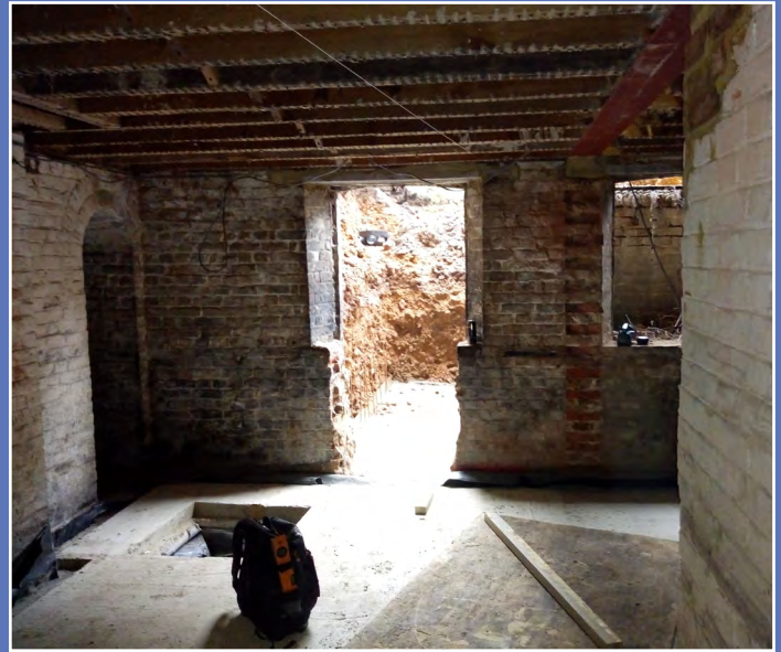
A new external doorway from the basement was also created
