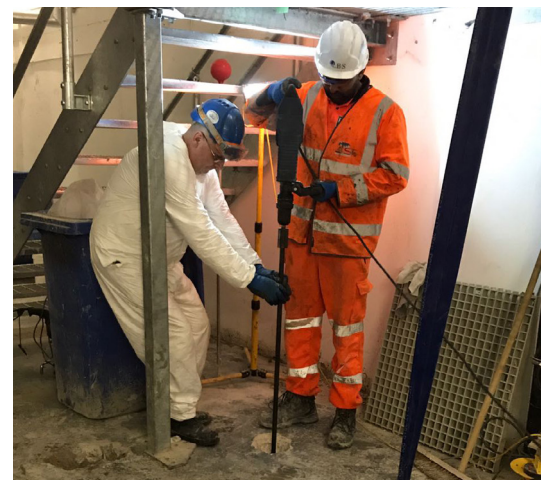
Packers were drilled into the slab to a depth of 2.5m.
