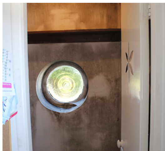
The pantry was severely affected by condensation.
