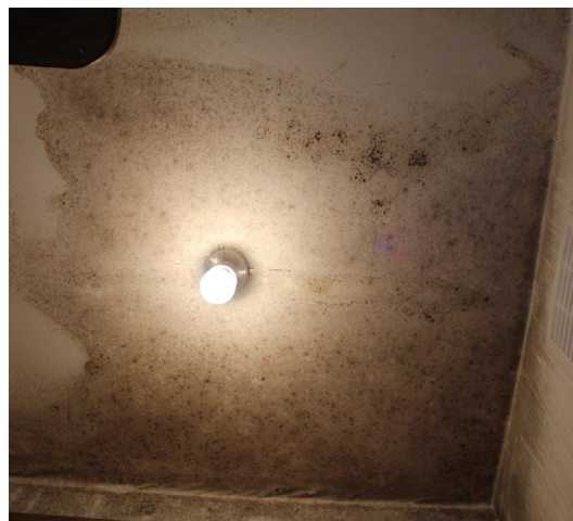
Black mould coated most of the walls and ceiling.
