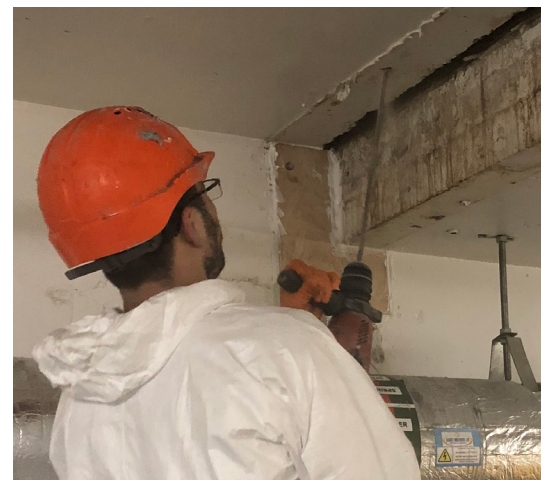
Drilling a hole for a 10mm injection packer.
