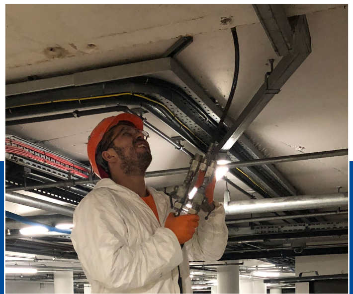
Injecting the 324-SR resin, done quickly and efficiently.
