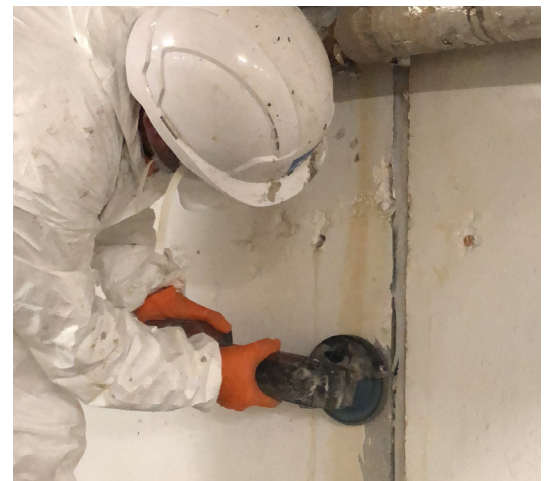
Preparing concrete to create a good key for FlexProof.
