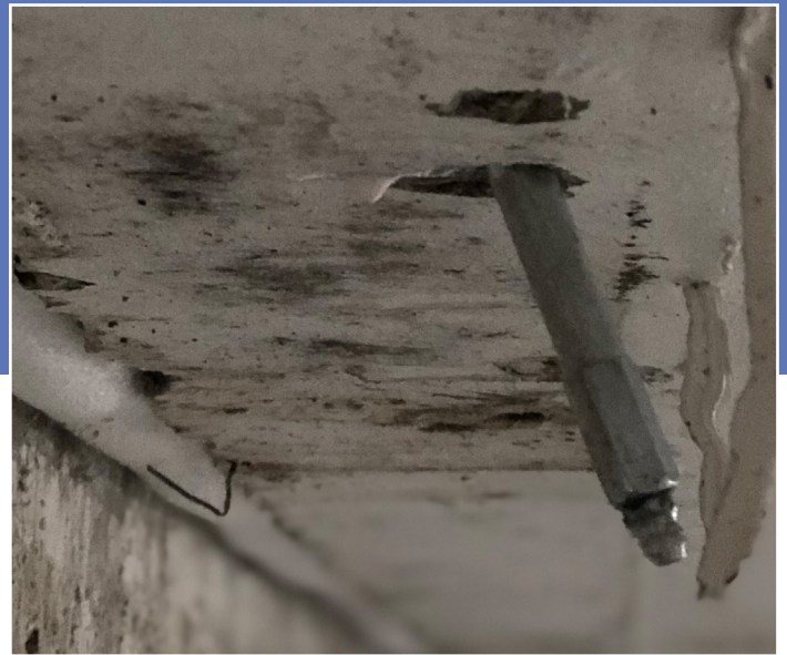
The packer is inserted behind the movement joint, ready to inject.
