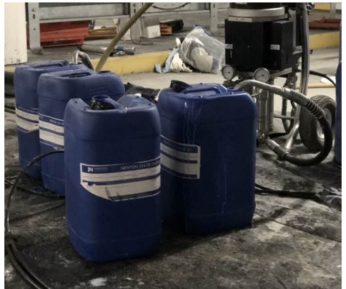
Newton 324-SR resin, ready to inject.
