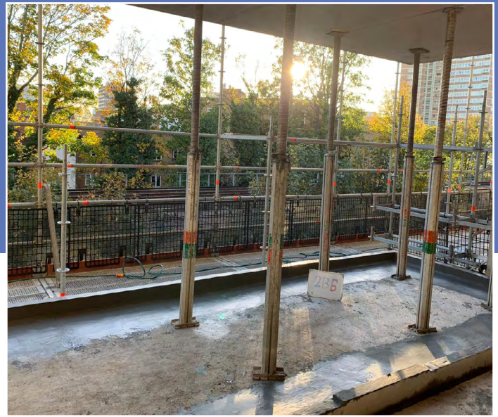
Formwork props prevented installation from occurring in one phase
