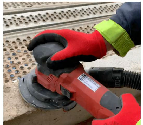
The concrete was correctly prepared before installation
