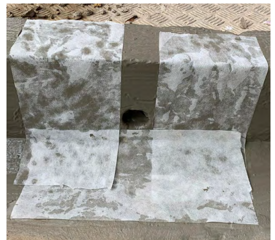
Newton 912-RT was used to reinforce the 103-S
