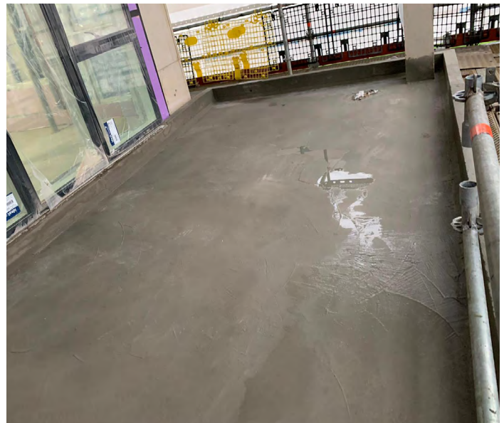
Arti returned to finish the waterproofing on a second phase
