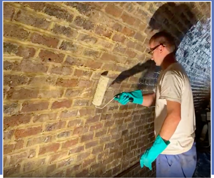
Newton 901-P was brush-applied in 2 coats over the course of 4 days
