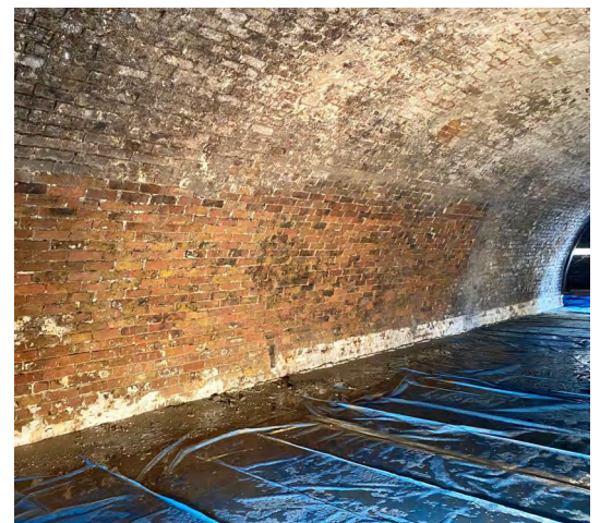
The brickwork needed thorough cleaning and repointing
