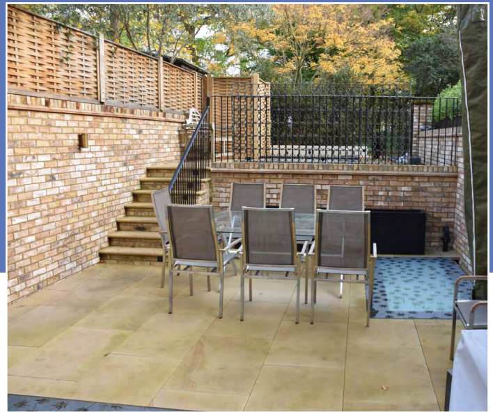
The completed rear deck with the new basement level beneath
