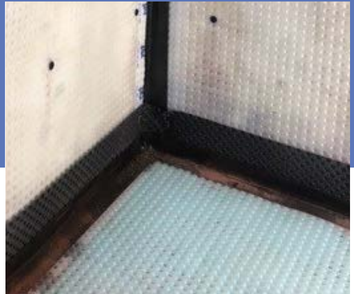
Floor to ceiling membrane fitting.
