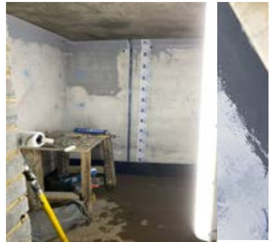
The client specified a waterproofed, habitable level.
