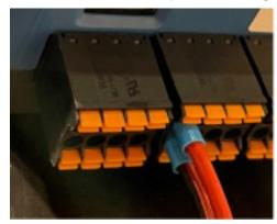
The terminals are designed to take both solid and stranded conductors. Bootlace ferrules can be added if preferred.
